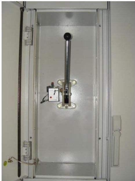
Figure 7.4 Position of the operating lever when the isolator switch-on
